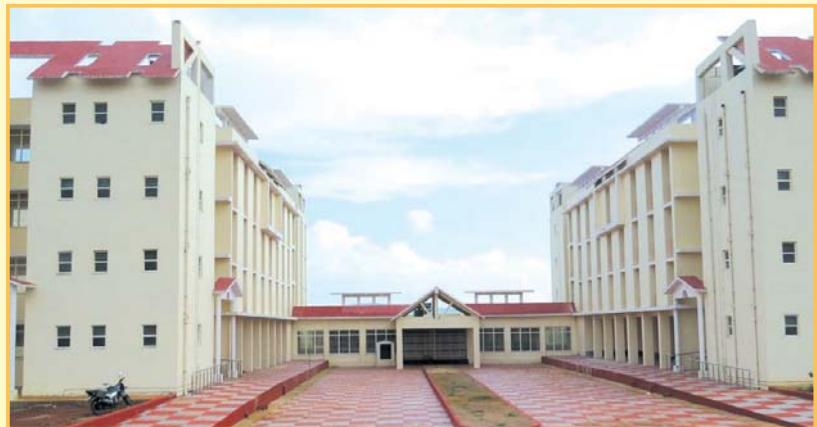
Close-up of Boys' Hostel at the permanent Campus of CUO, Sunabeda
