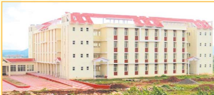
Girls' Hostel at the permanent Campus of CUO, Sunabeda
