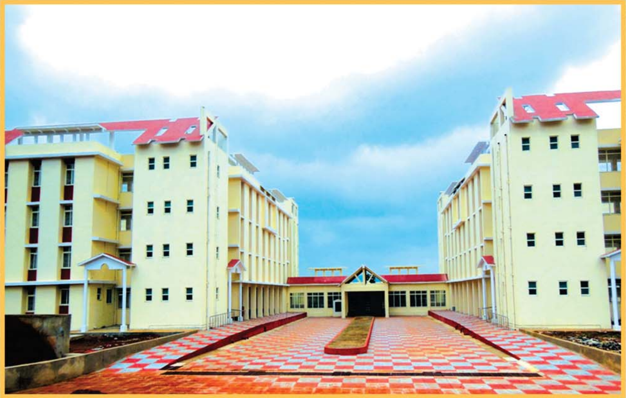
Boys' Hostel at CUO permanent Campus, Sunabeda
