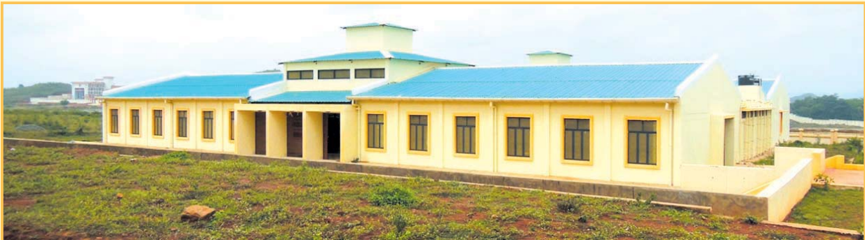
Pre-fabricated Academic Block at the permanent Campus of CUO, Sunabeda
