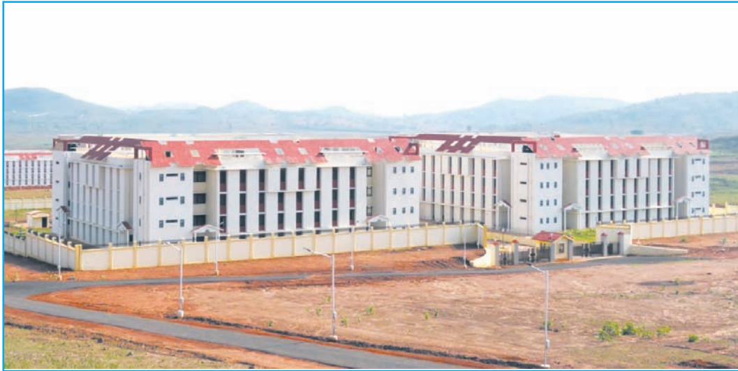
Girls' Hostel at CUO permanent campus, Sunabeda, commissioned.
