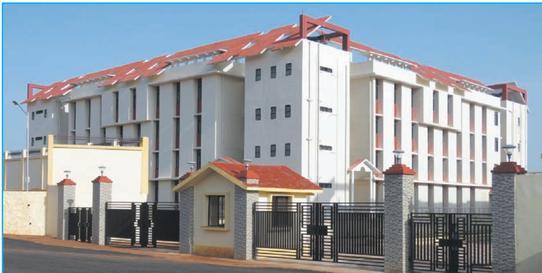
Boys' Hostel at CUO permanent campus, Sunabeda, commissioned.
